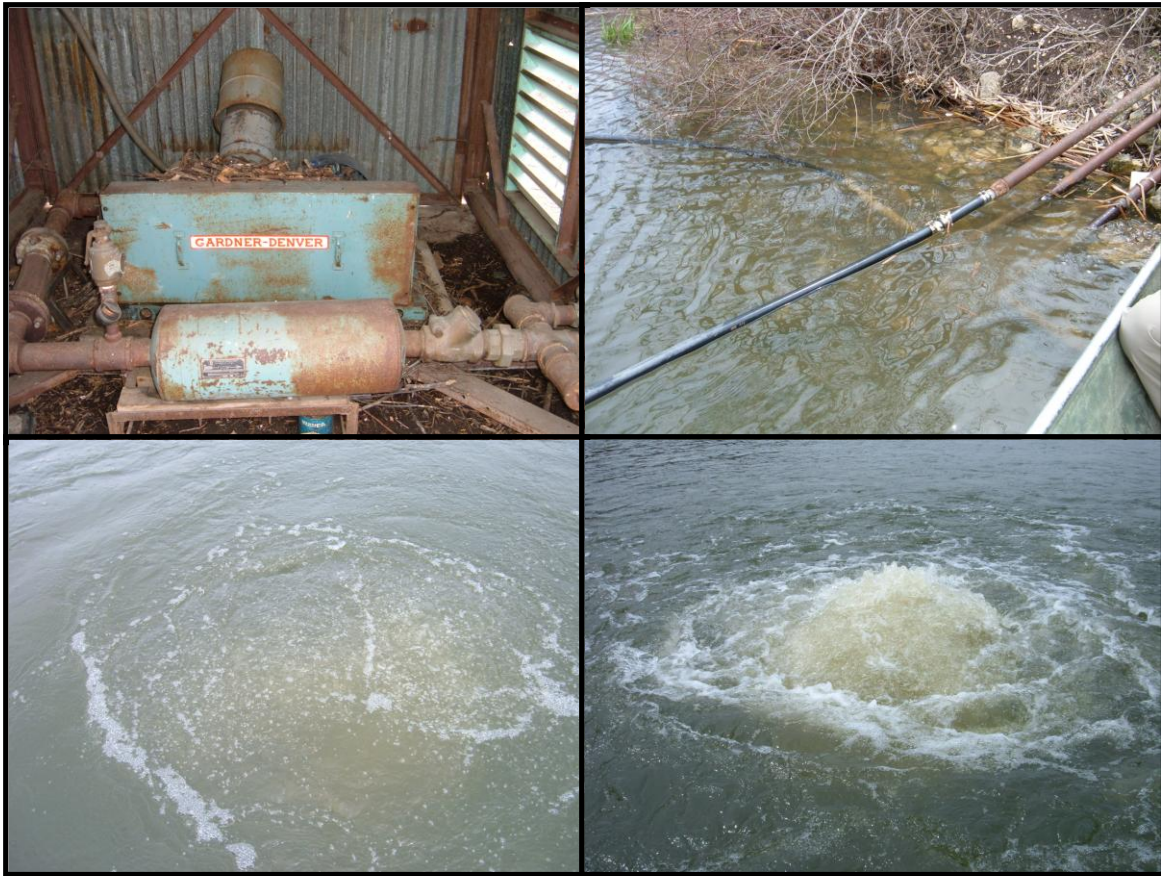
Figure 2. Pictures of destratification unit (top left); pipes to diffusers (top right); surface above two functioning Helixor diffusers (bottom).
